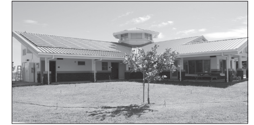
North Kohala Public Library's photovoltaic energy system panels can be seen on the left side of the roof.
